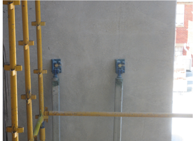
View of Prop foot attached to concrete panel
